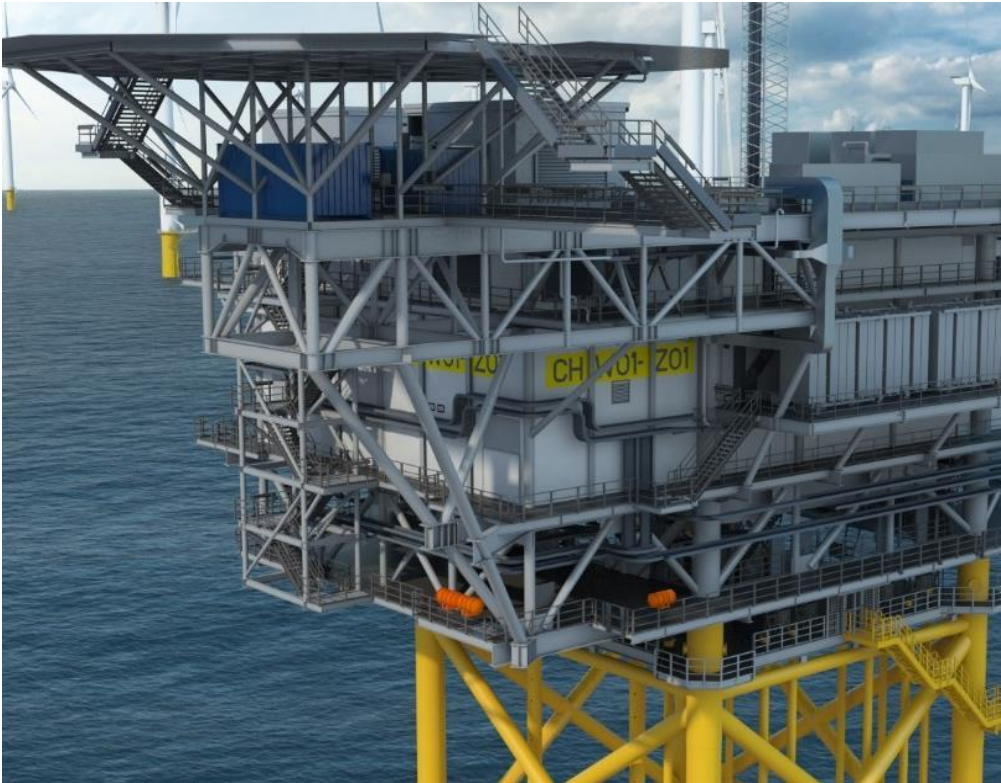
Figure 2.3: CGI rendering of the CHW01 offshore substation
