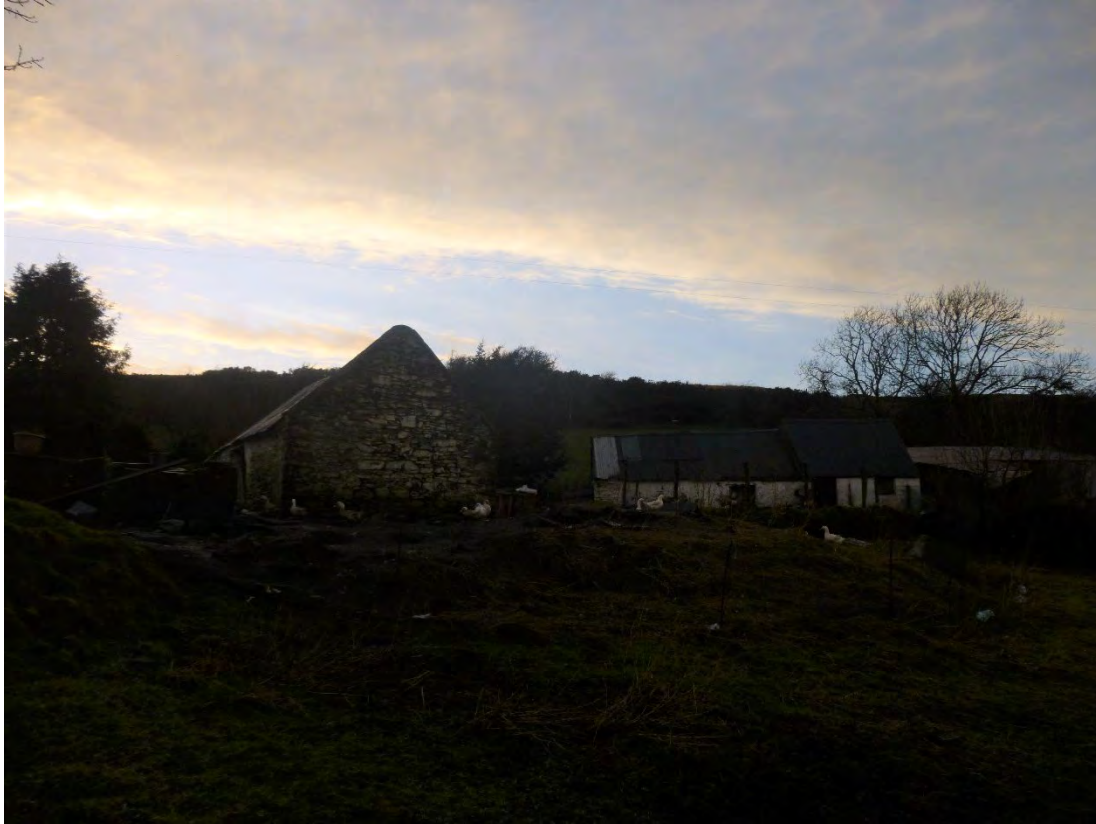
View towards CSA from assets along Meendamp Burn, east of Owenreagh Hill
