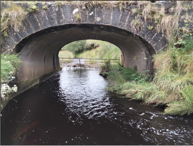
Plate 16: Road bridge over the Legnahone Burn
