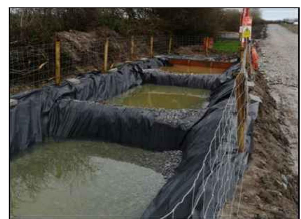
Completed Settling Pond System
