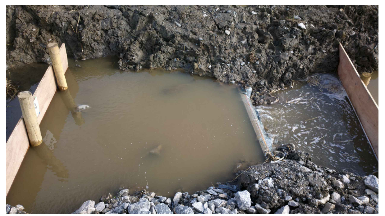
Baffle/Weir Detail
