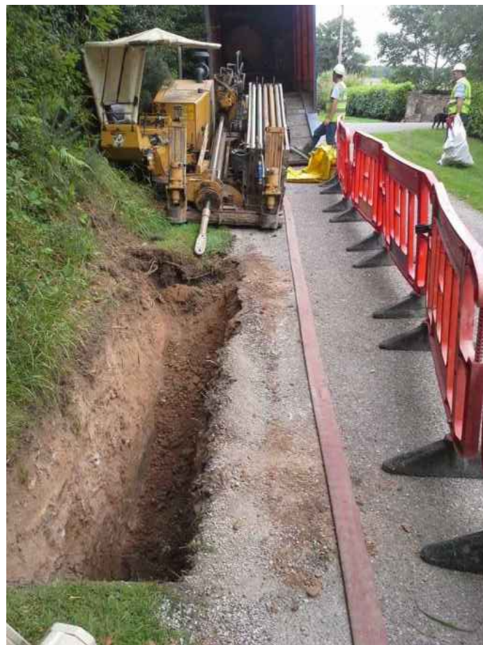
Drilling Rig/Launch Pit
