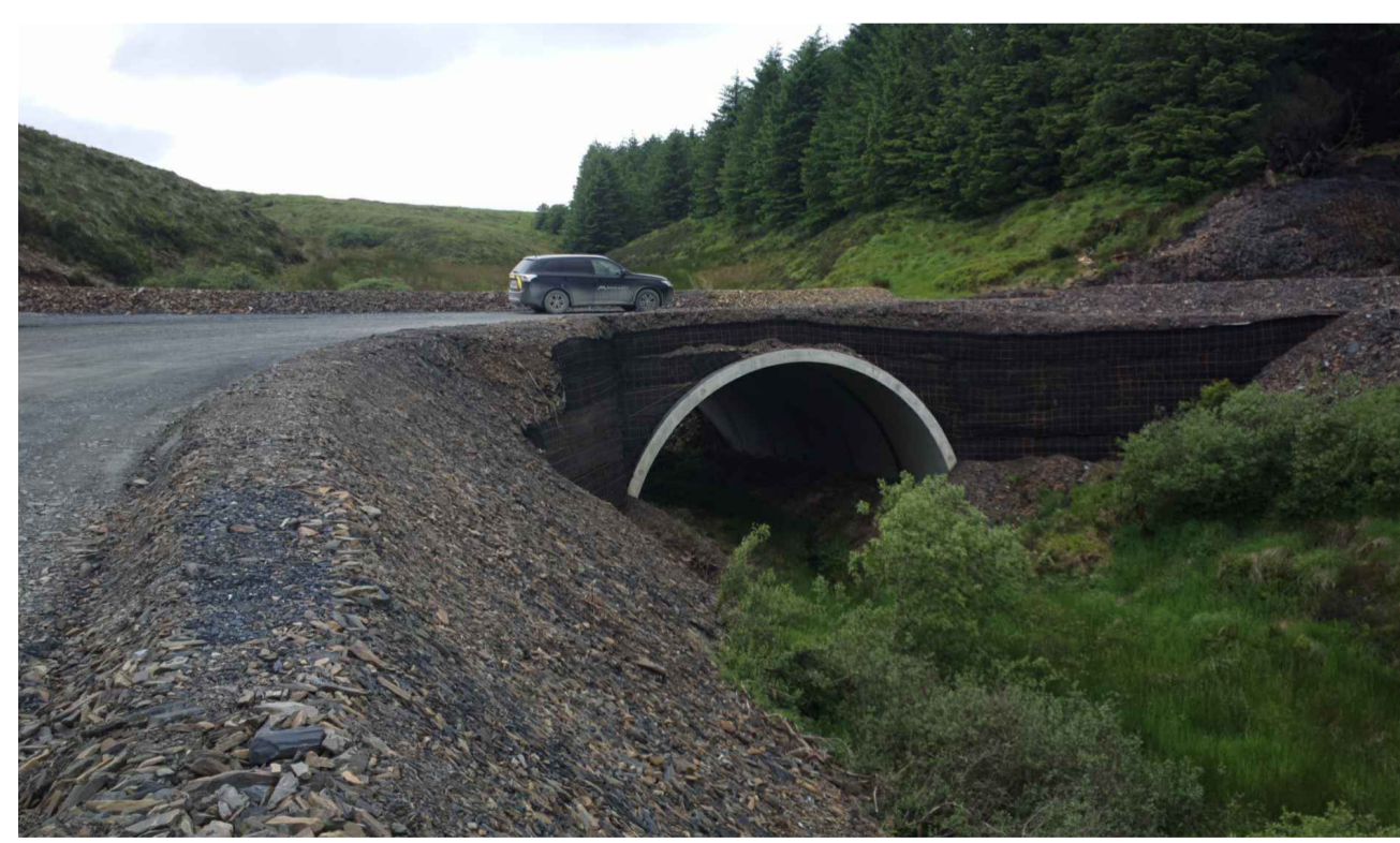
Bottomless Arch Culvert Crossing
