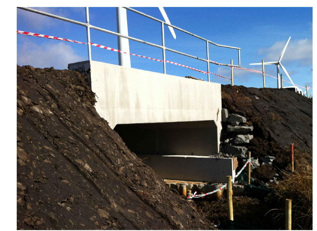
Bottomless Box Culvert Crossing
