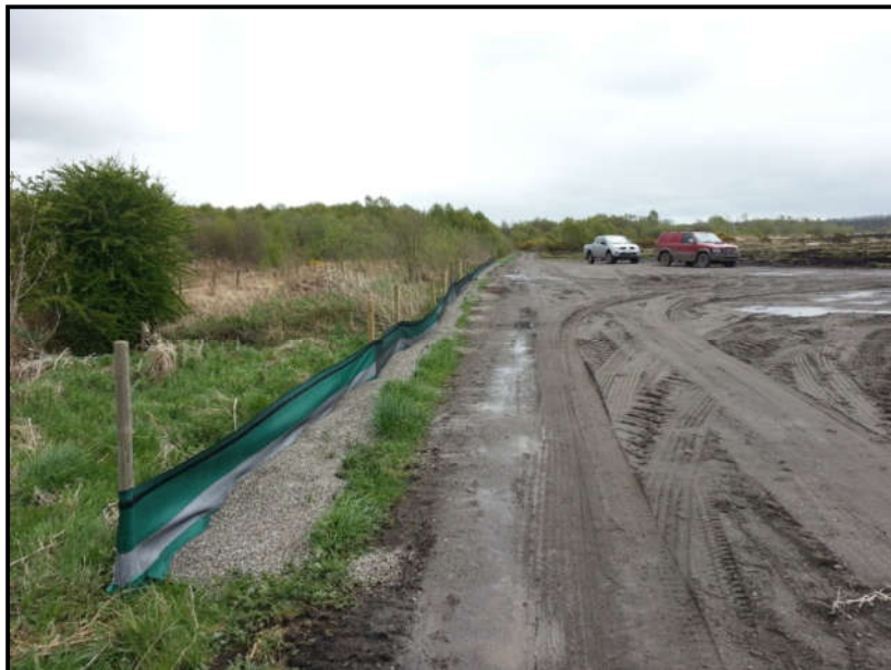
Plate 3-20: Example of a Silt curtain containment along existing tracks near watercourses
