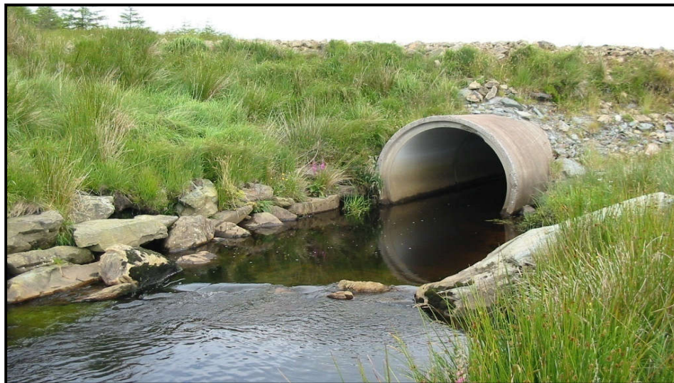
Plate 3-18: Example of a concrete pipe channel crossing
