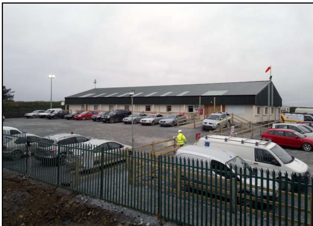
Plate 3-14: Wind farm example of the proposed temporary site construction compound
