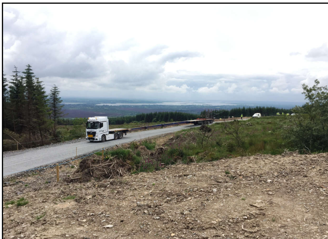
Plate 3-2: Wind farm site example of the proposed upgraded road
