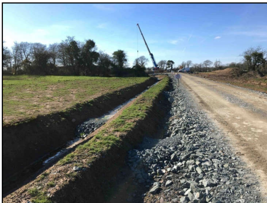
Plate 3-15: Wind farm example of the proposed Separation of Clean and Dirty Water Drainage Flood Attenuation
