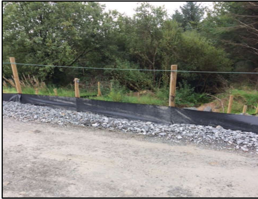
Plate 3-19: Example of a Dirty water containment at watercourse crossings
