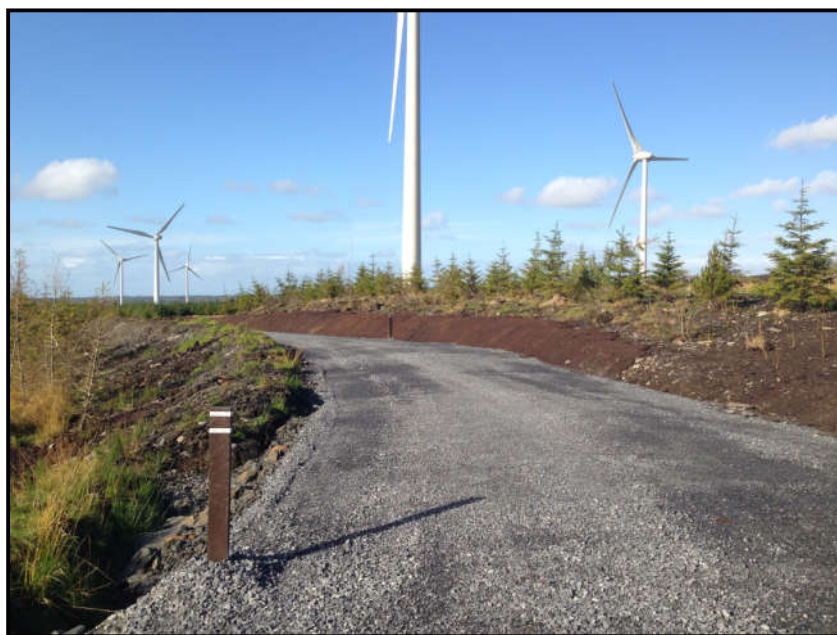
Plate 3-3: Wind farm site example of the proposed new founded track
