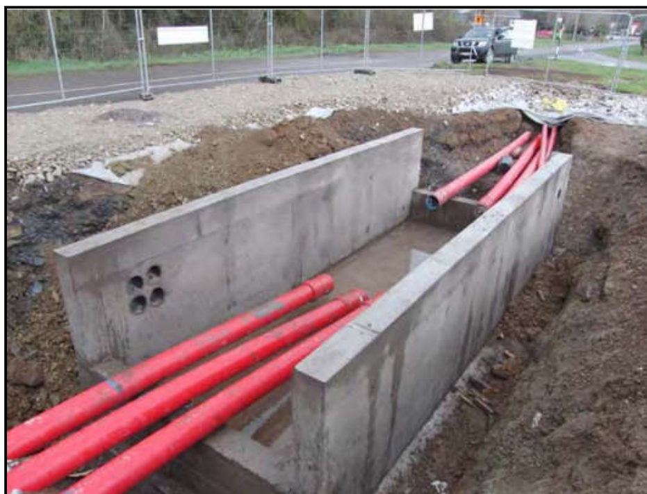
Plate 3-11: Grid Route example of the proposed joint bay construction
