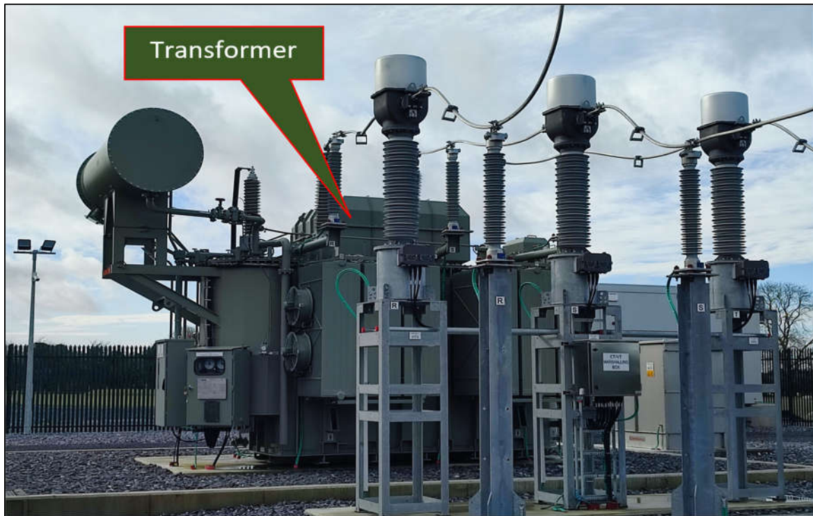
Figure 12-21. Indicative 110kV Transformer Unit.
