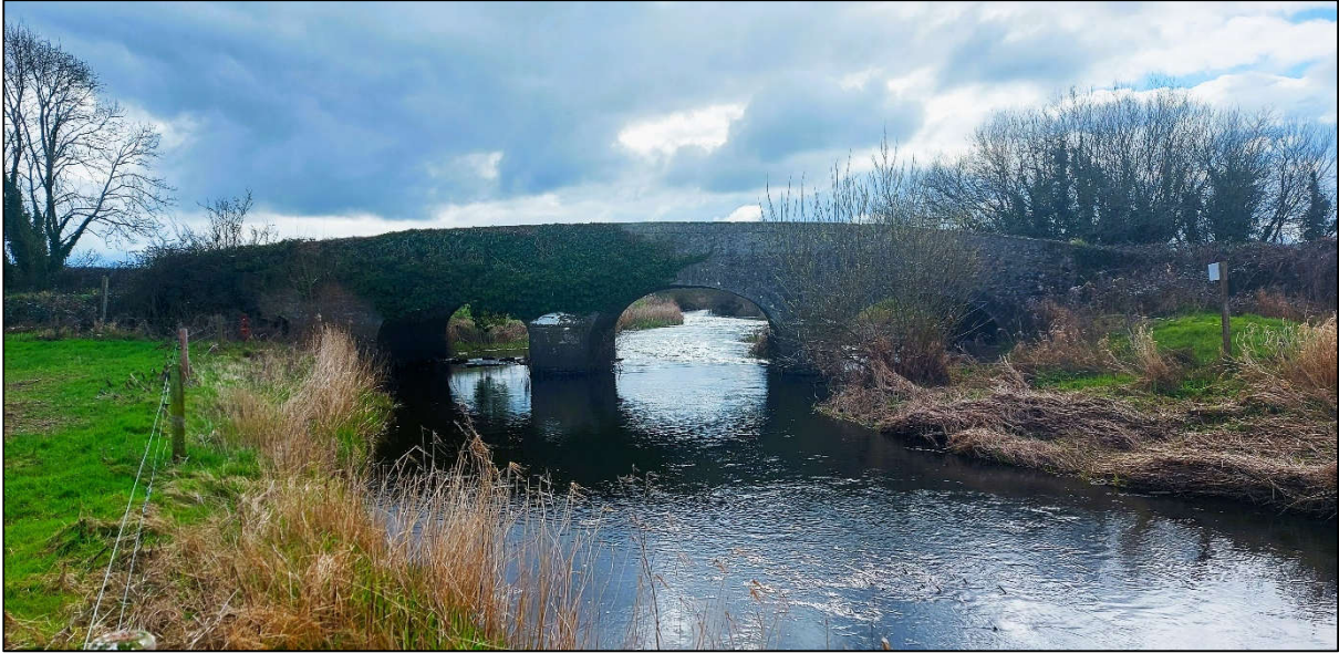
Figure 15-14: The Rossestown Bridge and River Suir
