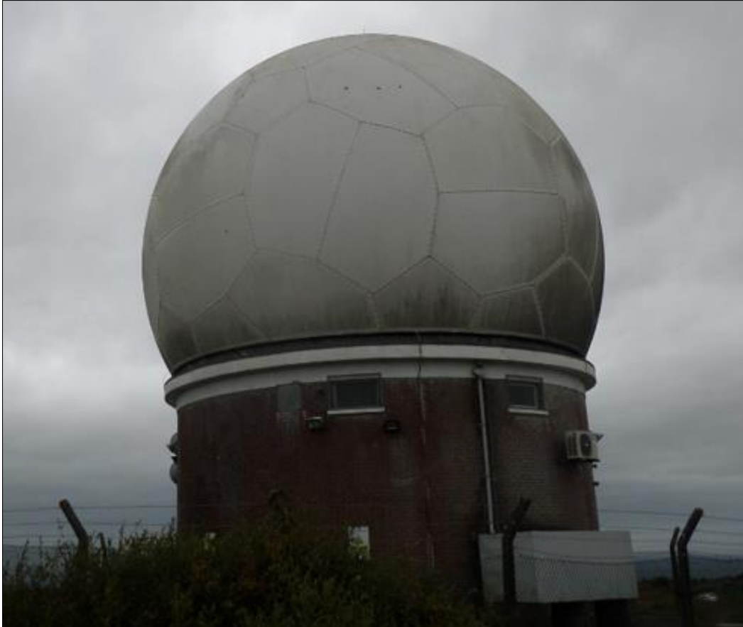
Figure 13. Woodcock Hill Radar Station
