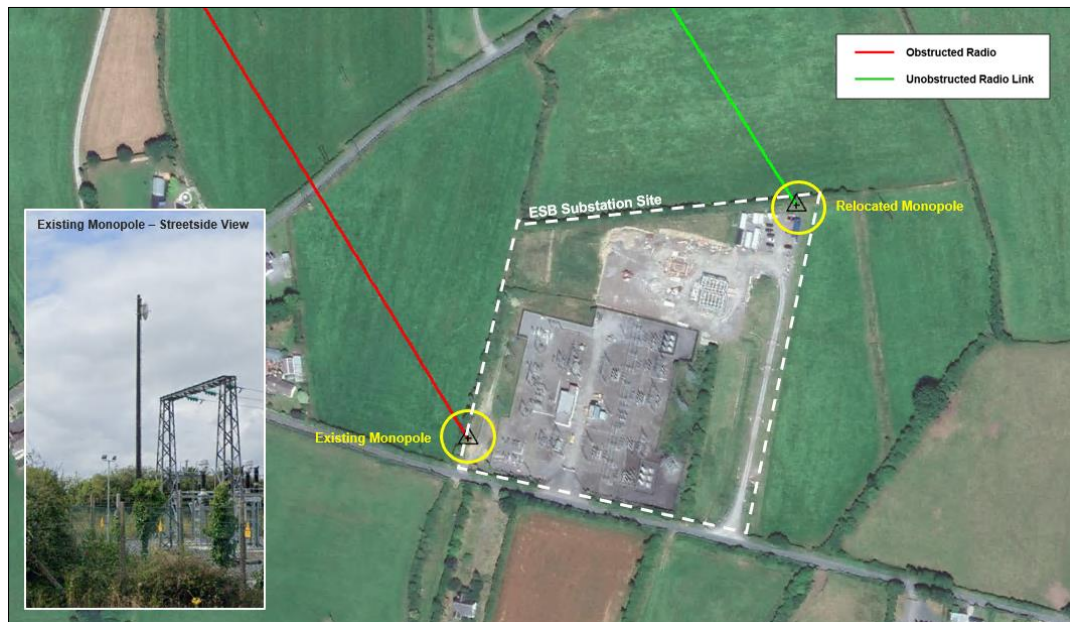
Figure 15. Relocated Monopole – Thurles 110kV Substation
