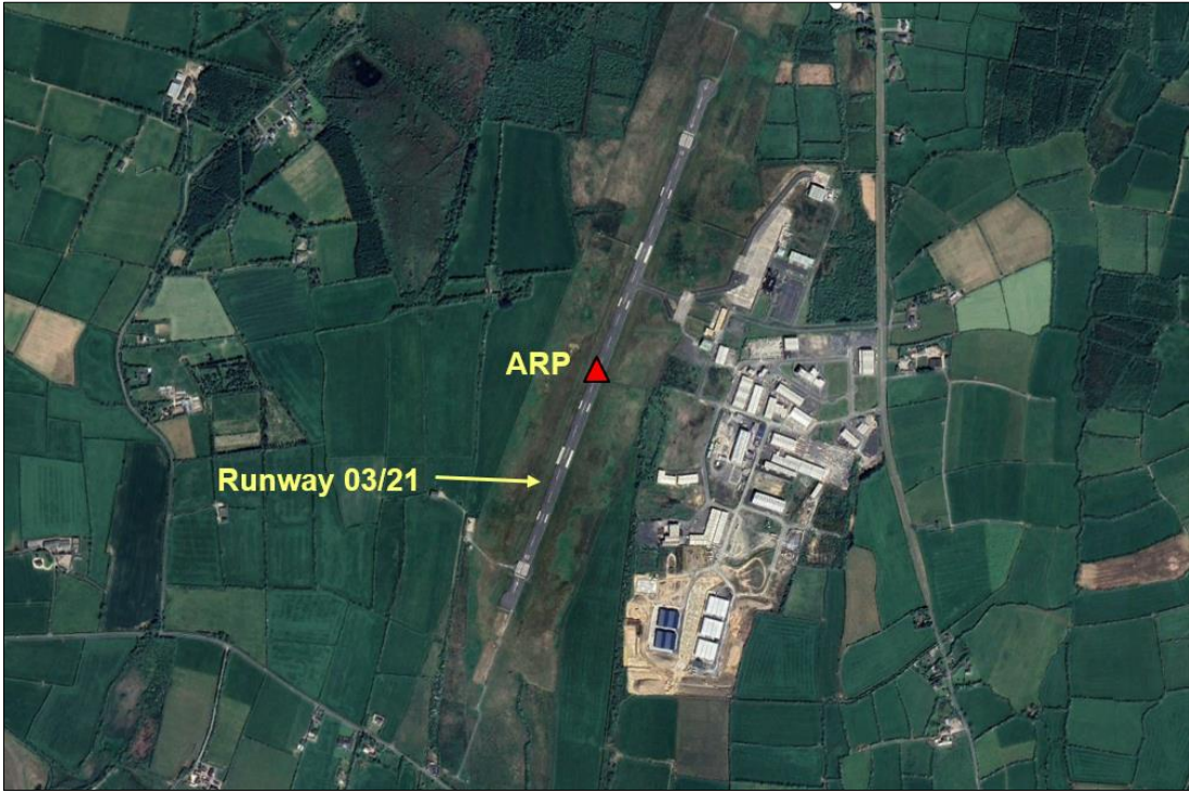
Figure 3. Waterford International Airport
