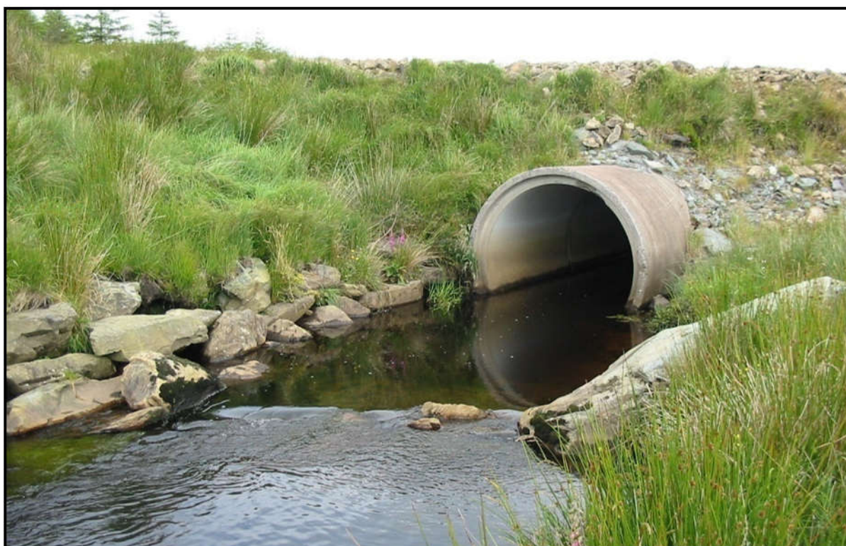
Figure 4-16: A concrete pipe channel crossing
