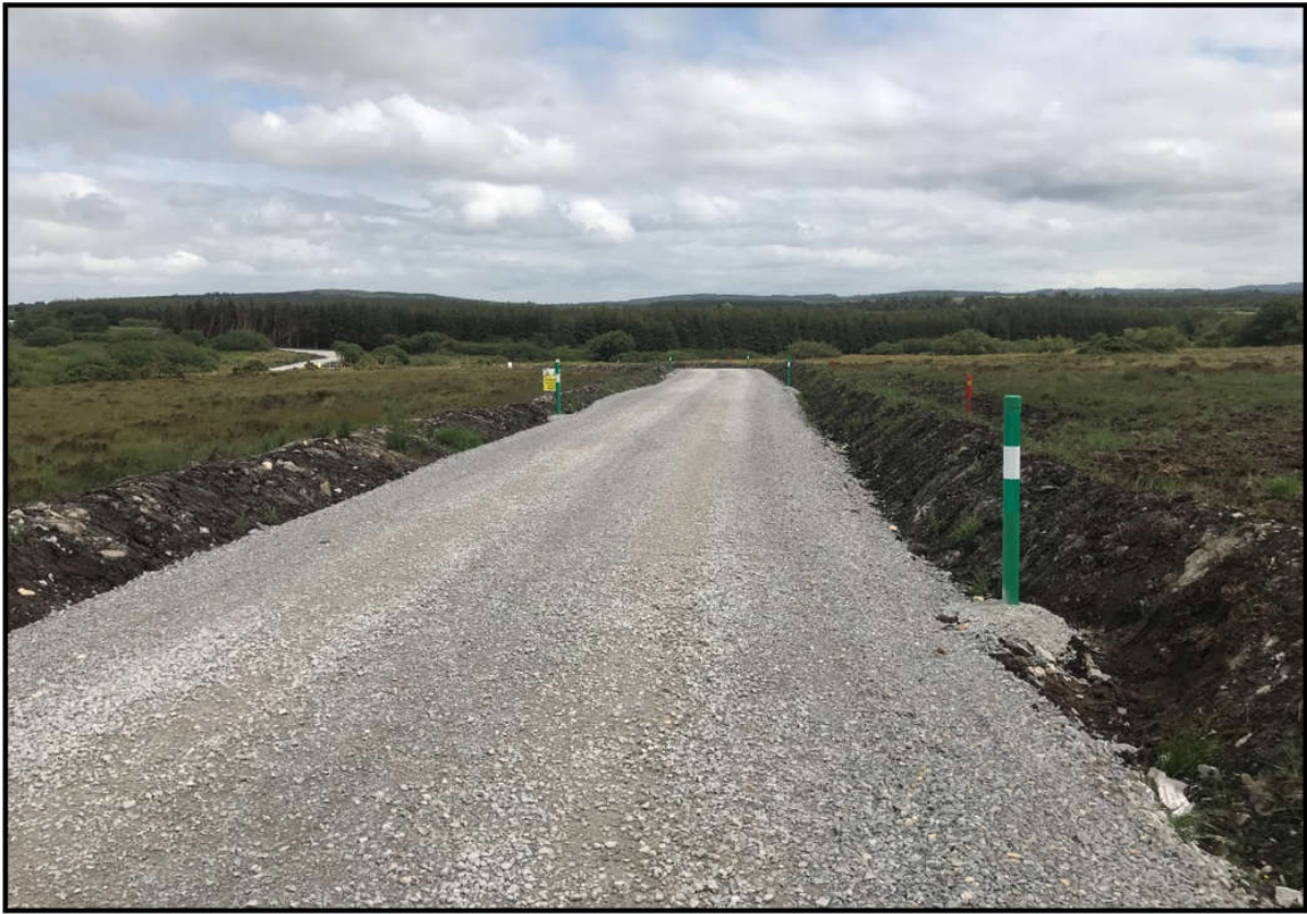
Figure 4-11: Floated road on a wind farm
