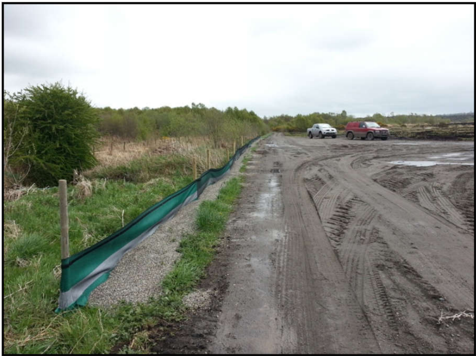
Figure 4-18: Silt curtain containment along existing roads near watercourses
