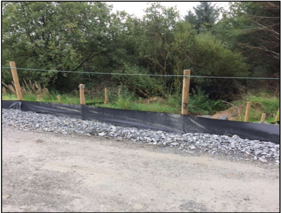
Figure 4-17: Dirty Water containment at watercourse crossings
