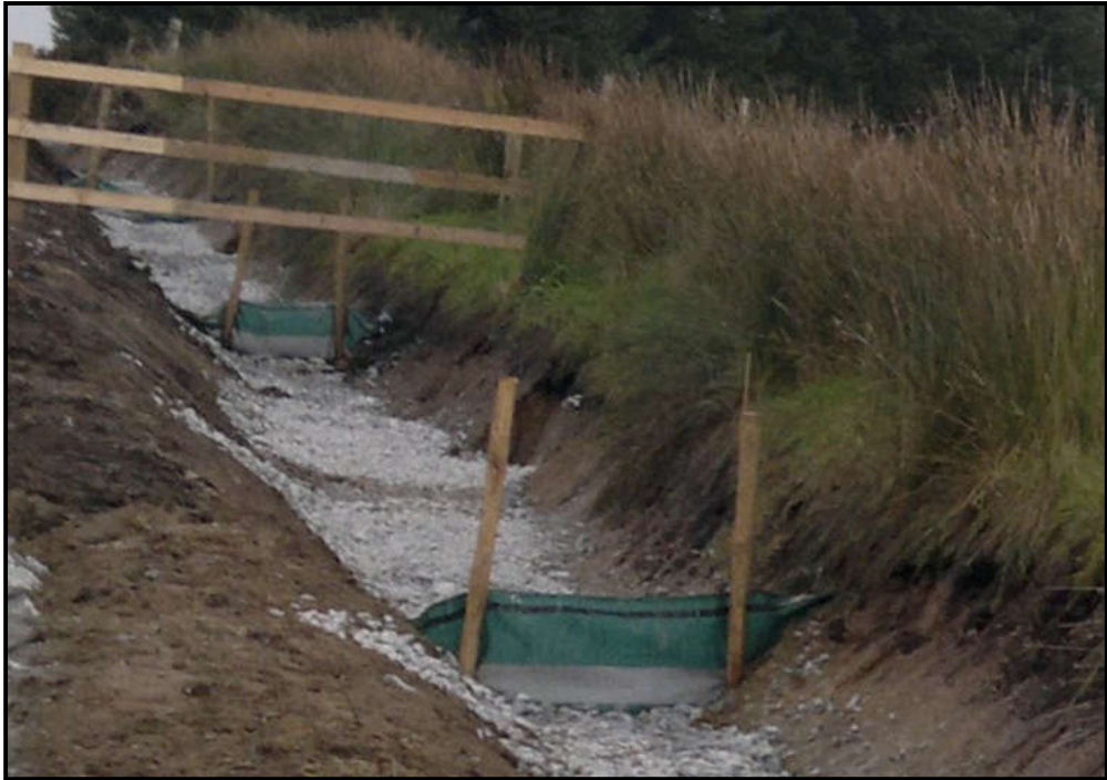
Figure 4-22 A silt fence used in conjunction with check dams along roadside drainage channels
