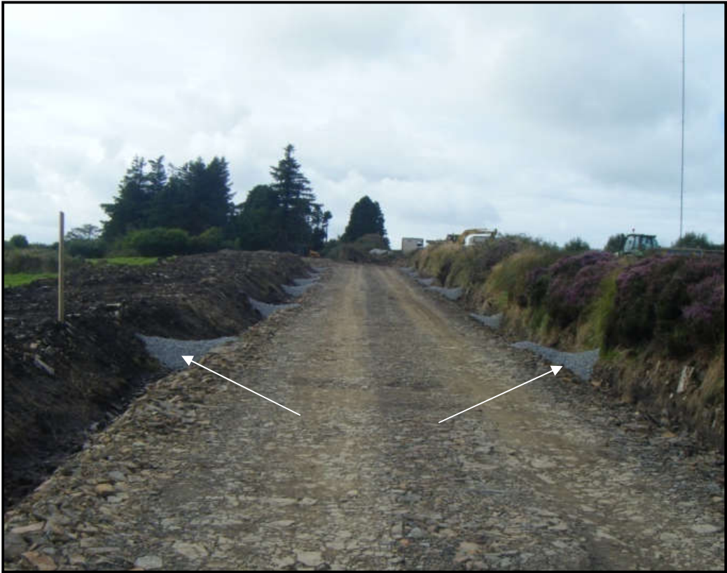
Figure 4-21: Check dams along roadside drainage channels
