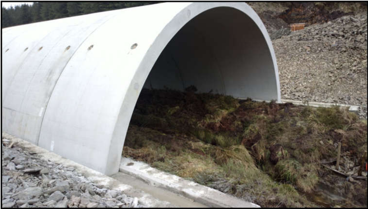
Figure 4-14: A clear span pre-cast concrete units in place over an existing watercourse
