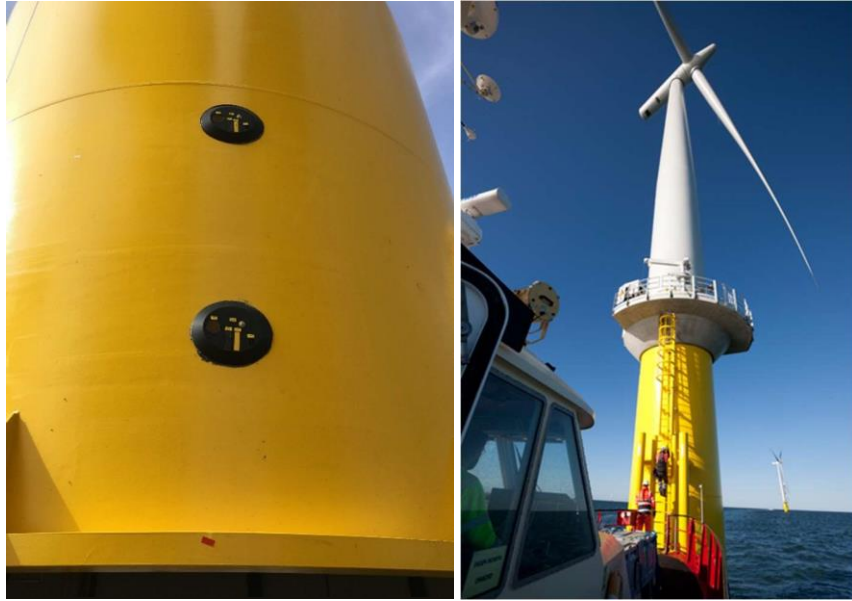
Figure 1 Transition piece with monitoring plates with probes installed to the left, to the right an offshore foundation with tower and turbine
