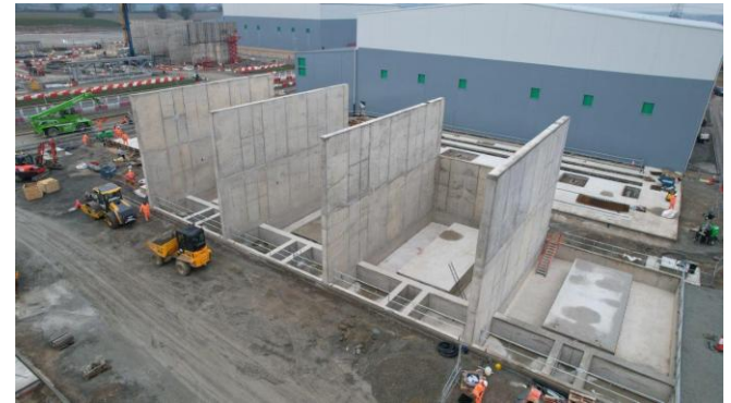
AC Yard, Cable Pits & Duct Installation
