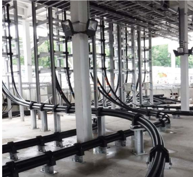
VolkerInfra are specialists in high voltage cable installation
