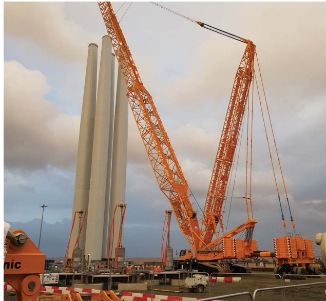
Pre-assembly of turbine towers Photo credit: Jamie Hampton
