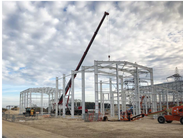
Steel frame under construction
