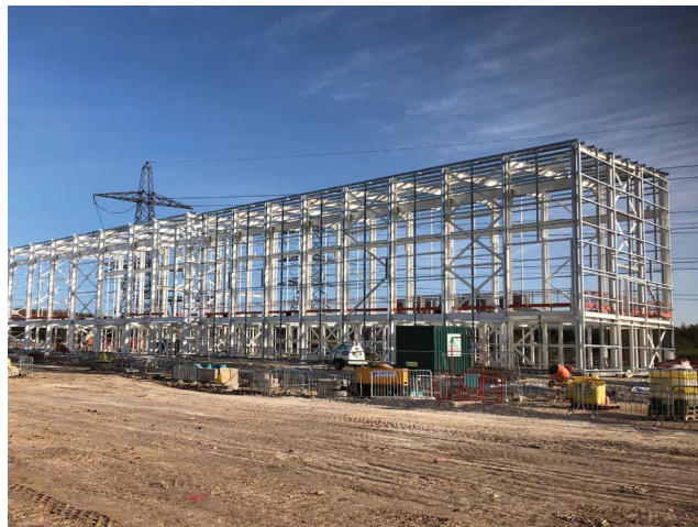
Skeleton of the switchgear building
