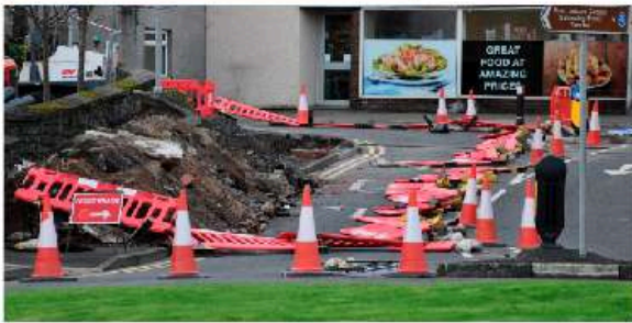
Above: works barriers blown over in Charlotte Street
