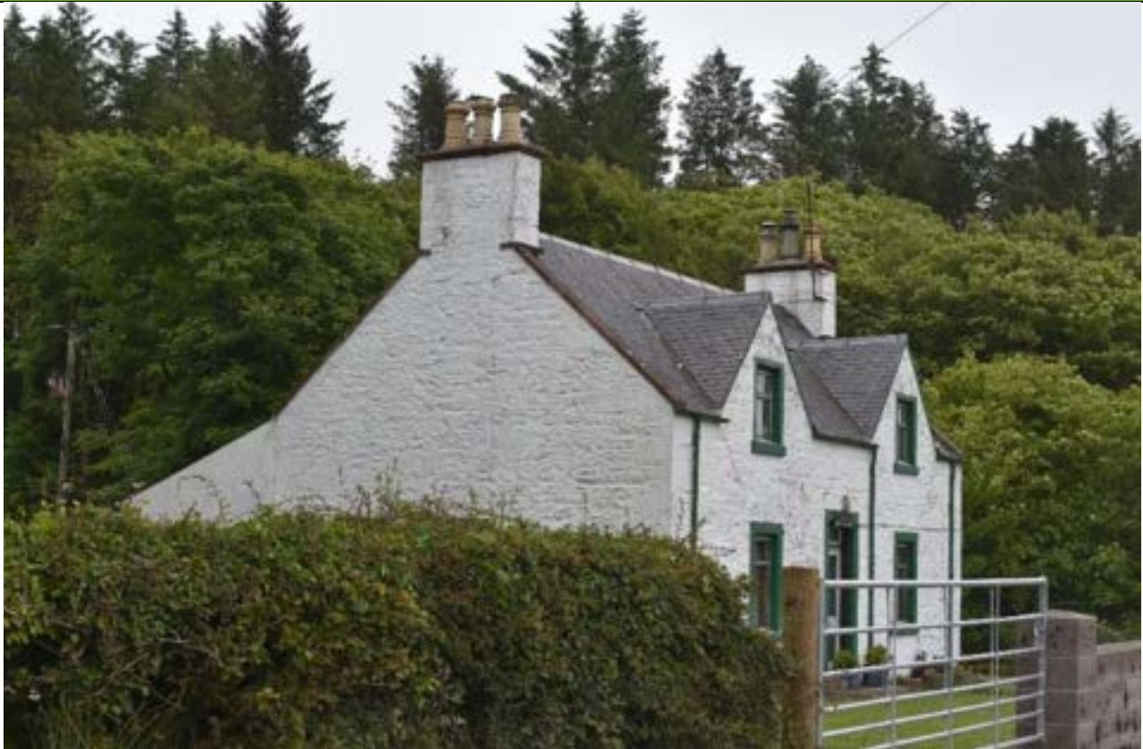
View of Burnbank from the north-west showing the primate south-western façade oriented towards the Proposed Development.
