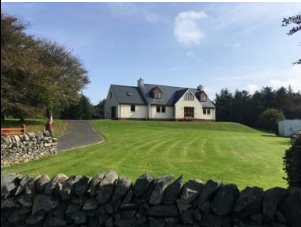
Cairnhapple House: View towards south-western facing façade.
